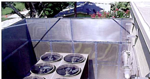
Panels prevented moving chillers
